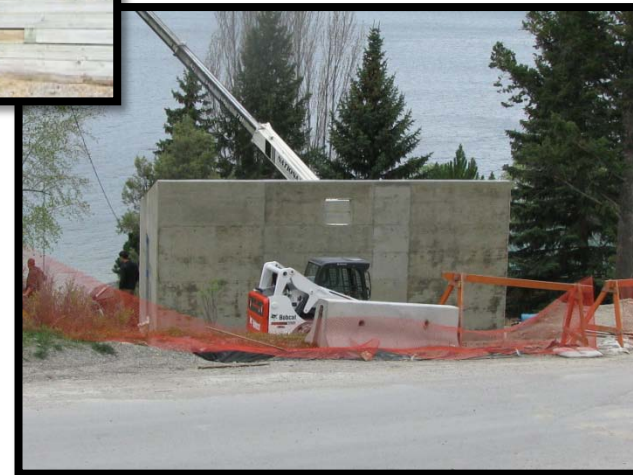
High Lift – under construction
