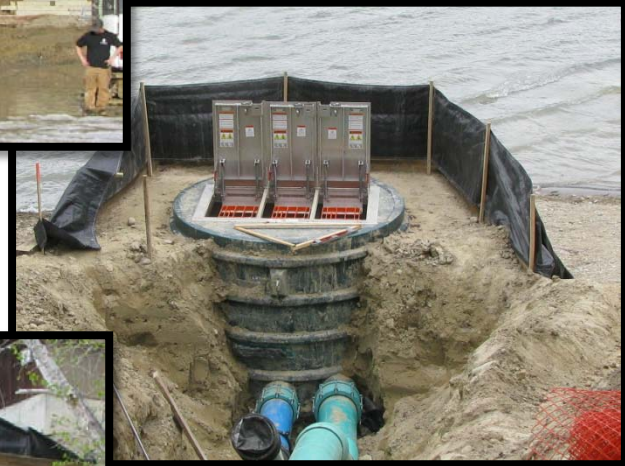
Low Lift – tank installed & retaining wall
